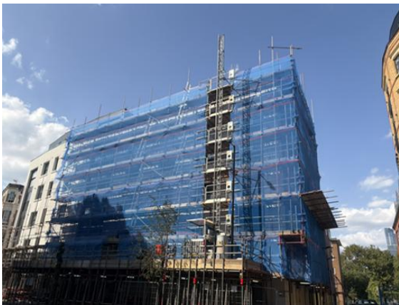
A photo of the Scaffold erection complete
