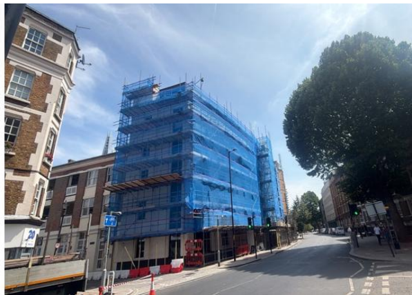
A photo of the Scaffold erection complete
